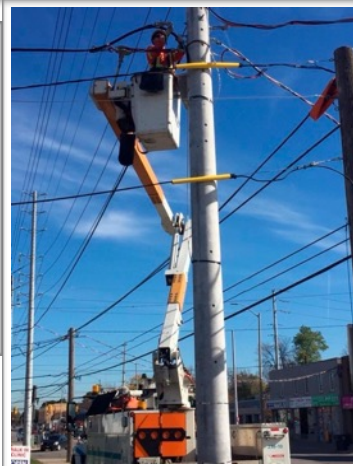
Enersource crews at work
